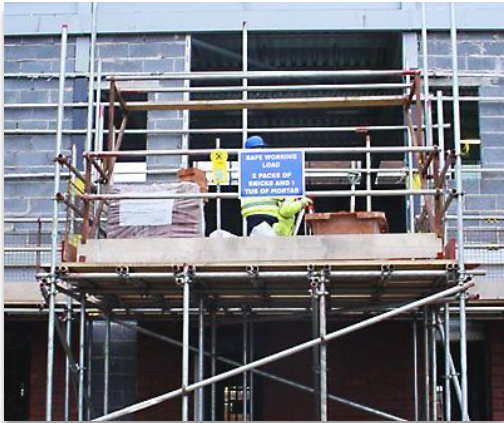
Components of typical loading bay gate
