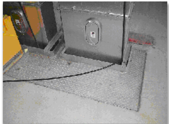
Metal Riser Flooring (with 65mm perimeter upstand)
