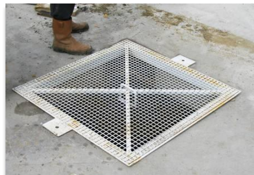
Temporary Cover (Awaiting permanent fixing to slab)
