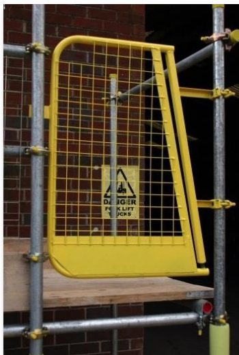
Proprietary Ladder Gate
