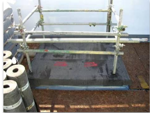
Typical Weatherproofed Roof Slab Opening
