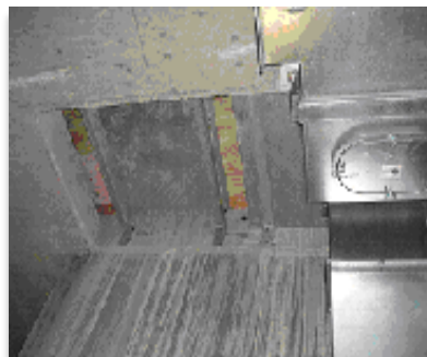
Metal Riser Flooring (with 65mm perimeter upstand)
