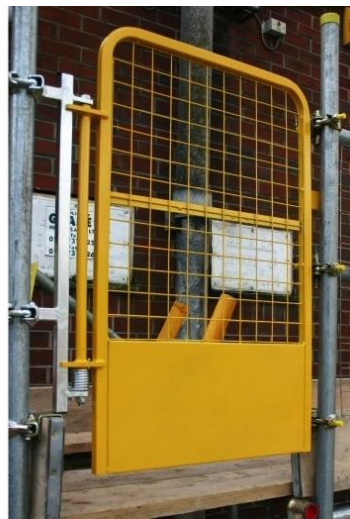
Proprietary Ladder Gate
