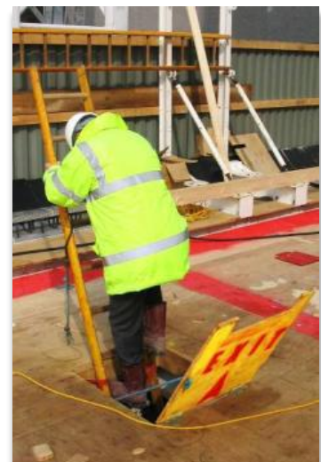
Ladder Hatch (note cutout)
