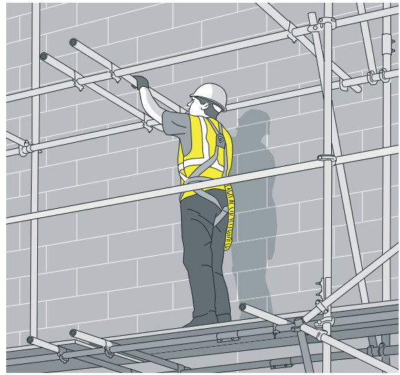
Figure 14 – Scaffolder working from a scaffolders working platform
